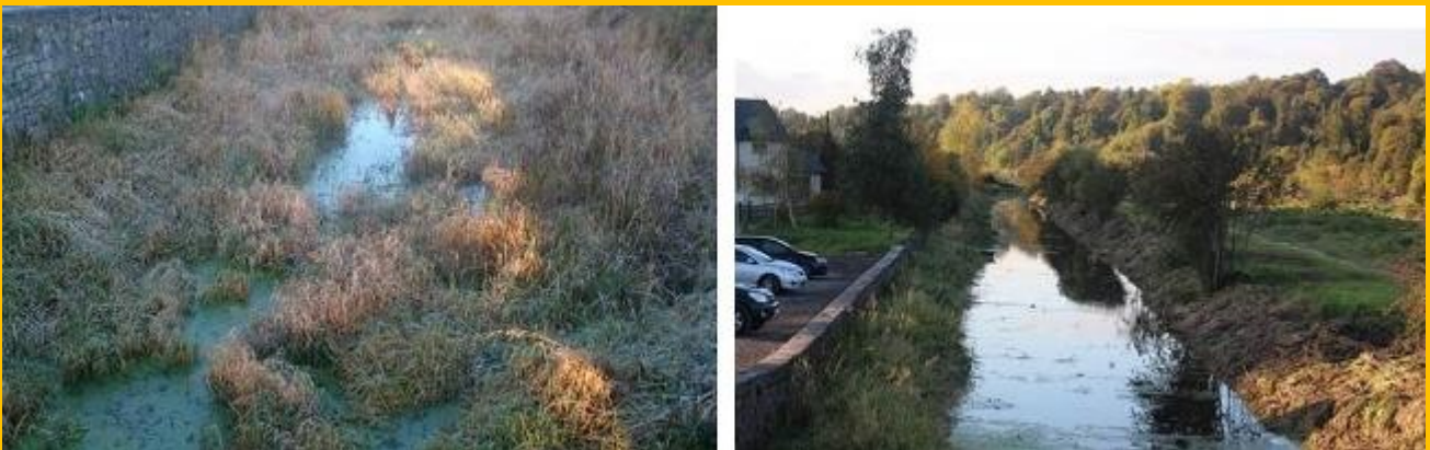
The Boyne Canal and Towpath Greenway, -Before and After
